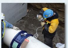
The Hymax 2000 offers an efficient range adjustable pressure assisted hydraulic sealing system. The gasket is compounded of an NSF 61 registered EPDM material.
