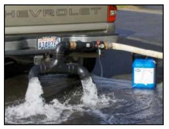
Typical Hydrant Flushing Application using the Truck Mounted Diffuser.
