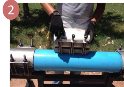
2 Loosen nuts to the end of the stud, place the clamp around the pipe centered over the break or damage area with the gasket flap at the top.
