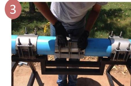
3 Tuck the gasket flap in place, close the fingers studs, engage the centermost stud(s) and finger tighten. NOTE: The clamp can be assembled beside the break and slid over the damaged area if the pipe surface and gasket have been properly lubricated.
