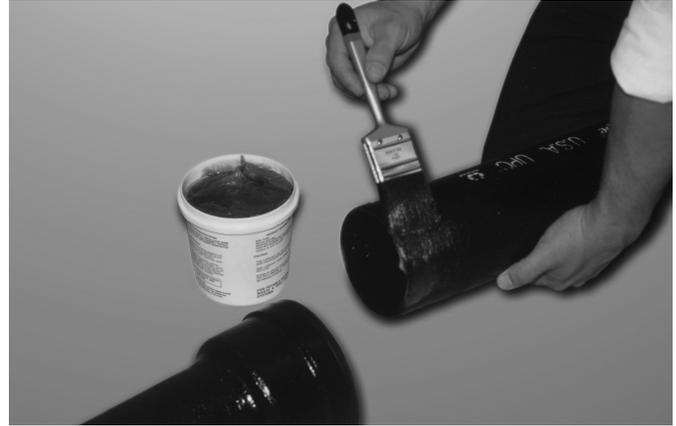
For large-diameter pipe and fittings (5" - 15"), we recommend that you use an adhesive lubricant.
