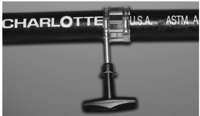
4. Slide the clamp assembly into position over the neoprene sleeve and use the following procedures to tighten to manufacturer's recommended torque requirements using a properly calibrated torque wrench:
