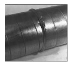
11. A completed, airtight, round transverse duct joint. Fast, neat and clean.
