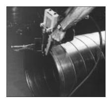
12" - 18" duct — 8" on center 20" - 28" duct — 12" on center 30" and larger duct — 18" on center
