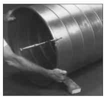
2. Seat flange permanently by pressing it so the leading edge of the duct is seated in the pocket of the flange and penetrates the sealant.
