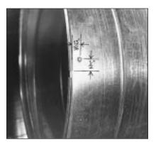
3. Begin securing the leg of the flange to the duct section by placing a pop rivet, screw, or spot weld within 1/2" of the end of the flange break. The fastener should be placed no closer than 3/4" or further than 1" from the face of the flange.
