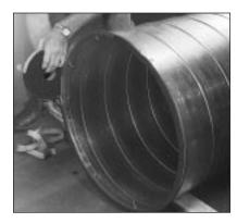
6. Complete the gasket application by installing Ductmate Neoprene gasket on the face of the flange around the entire circumference of **one** of the mating flanges.
