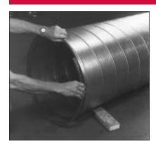
1. Start inner ring (flange) by inserting duct end into flange pocket at the break in the ring.
