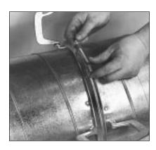
9. Slide closure ring over mating flanges and insert bolt.
