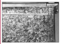
11. It is essential that the frame angle is fastened to the duct within 3/4" of the end of the angle at each corner
