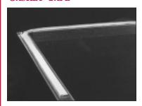
13. Start applying Ductmate 440 Gasket Tape about halfway between duct corners. Position gasket in center of Ductmate angle as in photo.
