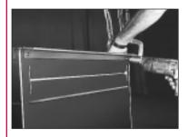
10. Work in one direction around duct when seating the frame. Fasten in sequence as you go. Do not fasten angle at corners first, it can cause seating problems.
