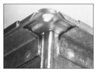
12. Ductmate angle may be fastened to the duct with self drilling screws or spotwelds.
