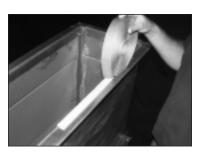
\*13A. Start applying Ductmate 440 1" x 3/16" Gasket Tape about halfway between duct corners. Position gasket to the inside edge of the Ductmate angle as in photo.
