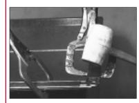
8. Use a mallet to seat the frame onto the duct. Establish metal to metal contact along length of the angle.
