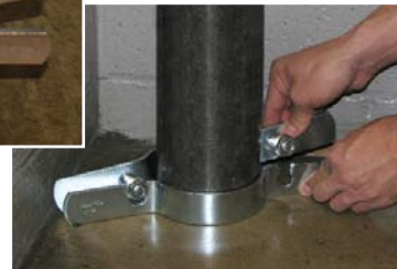
2. Hold bolt in place while aligning clamp
