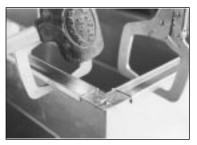
7. Use a mallet to seat the frame onto the duct. *Establish metal to metal contact along length of the angle.*
