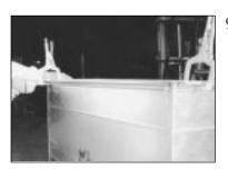
Work in one direction around duct when seating the frame.
