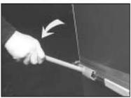
**WITH DM440 GASKET** For all low, medium and high pressure applications, use 6" cleat, 24" O.C.
