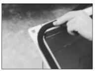
3. Position Neoprene gasket in an arc so that it covers the three points in the duct corner. Gasket must cover all three points.
