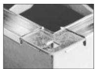
8. The duct must be seated all the way into the WDCI angle in order to penetrate the integral mastic sealant and avoid leakage.
