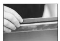
Apply Neoprene gasket completely around WDCI frame to the beginning point. Butt the two ends of the gasket up against each other. Do not overlap the two ends.
