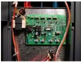
1. **Zone wiring and troubleshooting convenience** – the addition of the zone board (fits within basic boiler cabinet) allows for easy terminal block and point to point wiring for each zone thermostat and each zone valve.
