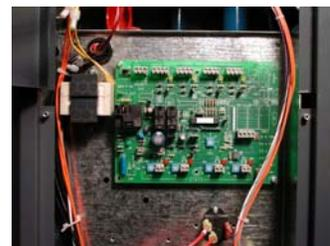
1. **Zone wiring and troubleshooting convenience** – the addition of the zone board (fits within basic boiler cabinet) allows for easy terminal block and point to point wiring for each zone thermostat and each zone valve.
