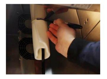
Install the Air Scoop Kit. Start by removing the upper set of screws located above the fan on the back wall of the cabinet
