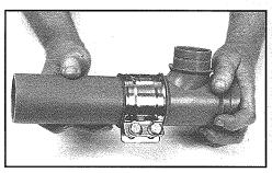
**STEP 2**Position stainless steel band so equal amounts of inner material show on each side of band.
