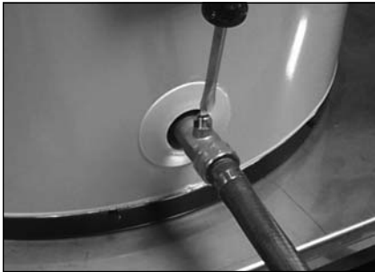
Draining the old water heater.
