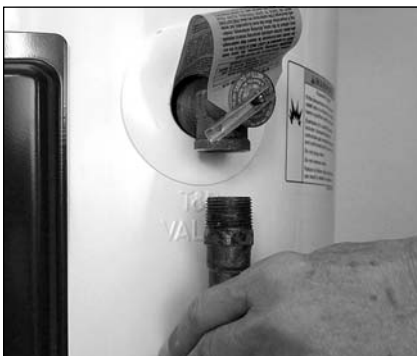
Removing the T&P Relief Valve discharge pipe.
