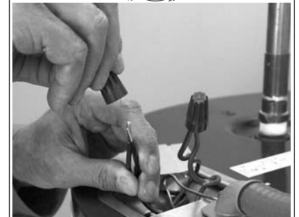
Connecting the electrical wires.
