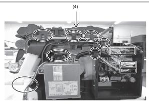
(5) Fasten the earth wire (green) in the communication box together with the earth wire (green) on the board of the control box as shown below and in the bottommost figure of the previous page.
