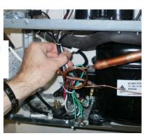
Tee and tube to Versafiller are packaged with PWSBF unit. One branch of tee will supply valve on dummy unit. Other branch of tee will connect to Versafiller. **Note:** "Versafiller ready" single units do not use tee since water line from cooling tank only supplies water to bottle filler.
