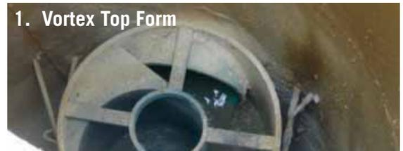
Wastewater flows into the Vortex Top Form directing the flow around a channel of decreasing radius. At the same time, the Vortex channel slopes downward to accelerate the wastewater to a supercritical velocity.
