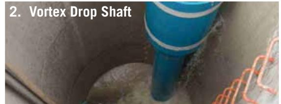
Once in the smaller Drop Shaft, the velocity and centrifugal forces generated cause the flow to hug the inside walls of the Drop Shaft. This spiraling flow creates a negative air core, drawing airborne gases down to the Energy Dissipation Pool.
