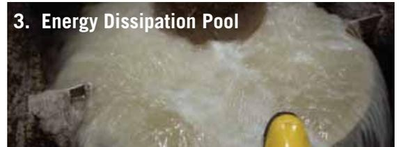
The flow exit is submerged in the Energy Dissipation Pool at the bottom of the Vortex. Air and gases drawn down the air core are forced back through the wastewater and re-entrained into the flow. This significantly increases the dissolved oxygen concentration, and the odorous compounds are quickly oxidized.
