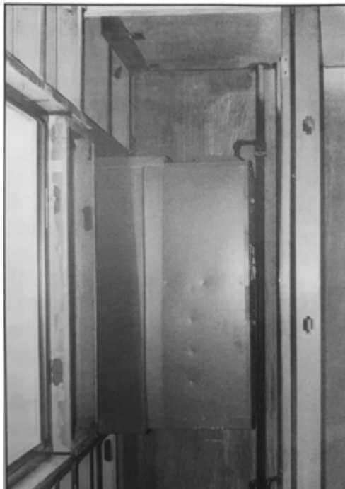
Figure: 29: Wall sleeve fastened to steel 2" x 4" studs with screws fasteners shot through sides of wall sleeve.
