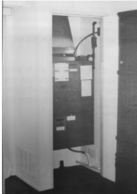
Fig. 32: Return grille with direct opening into equipment room allows sore to escape into living area and should be avoided. Also note lack of unit support at bottom
