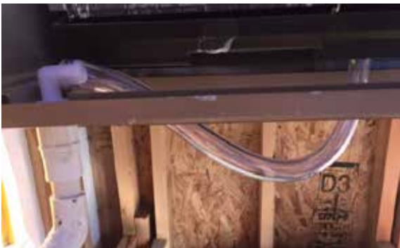
Figure 34: Inside of unit at return-air duct flange, showing sealed condensate tube opening
