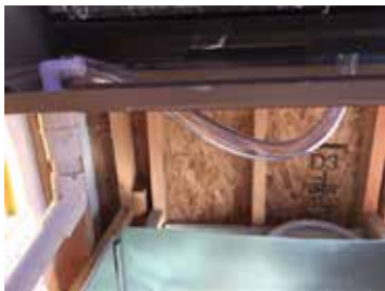
Figure 21: Condensate-tube installed
