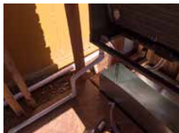
Figure 22: Condensate-tube installed
