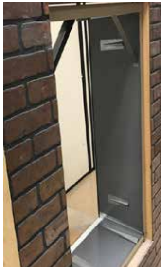
Figure 13 - Fasteners shot through wall sleeve sides into back wall
