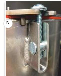
The SL 40-399G3 features a new and innovative side bolt heat exchanger lid configuration.
