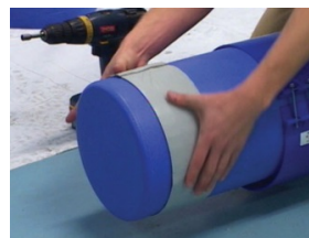
Tack gasket down and apply pressure
