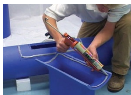
Continuous 3/8" sealant bead.
