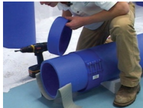
Tack gasket halfway around duct
