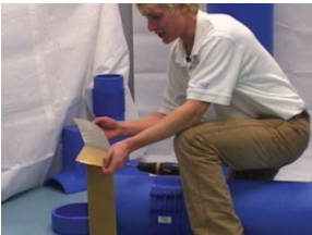
Peel off gasket backing
