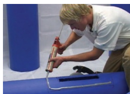
Continuous 3/8" sealant bead.
