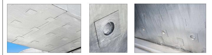
On ducts over 24" (60 cm) in width, pin bottom on 12" (30 cm) centers. Cover pins with a 3" (8 cm) square minimum of FlexClad.
