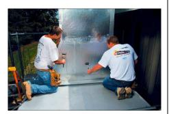
Roll entire surface firmly with a hand roller to ensure good adhesion.
