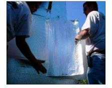
Pull release film from behind membrane and continue to press into place.
