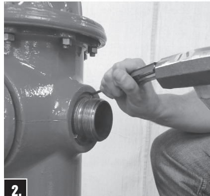
2. Remove stainless steel Nozzle Lock by driving it out with a pointed tool and hammer.
