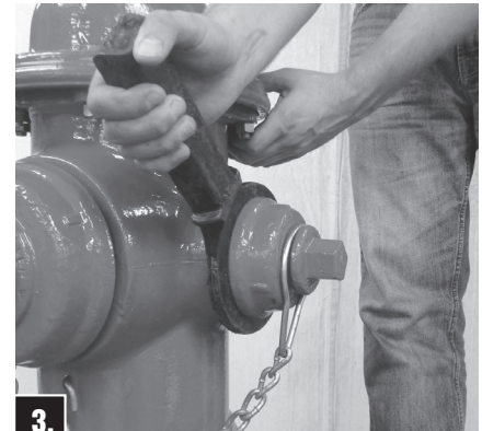
3. Place Nozzle Wrench, A-316, on Nozzle with Wrench Forks facing toward Hydrant Barrel and locked onto Nozzle Drive Lugs. Replace Nozzle Cap and tighten until Cap rests loosely against backside of Wrench. Remove Nozzle (nozzle threads out in a clockwise rotation). Additional leverage may be obtained by placing a length of 2" schedule 40 steel pipe over the handle of the Nozzle Wrench.
