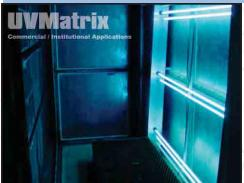
The UVMatrix SI-Series uses UVC light to disinfect HVAC coils in large air handlers. The benefit is improved indoor air quality (IAQ) and clean, efficient HVAC operation with reduced maintenance and energy costs.
