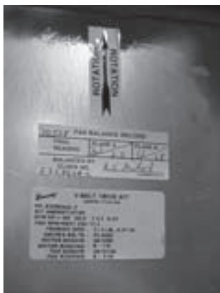
Figure O-M-7. Location of fan belt label on fan scroll.
