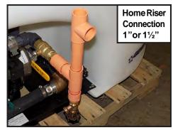
Thread the riser into manifold and tighten until riser is in an upright position.
