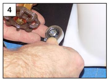
Install the bolts on both sides of base plate.
