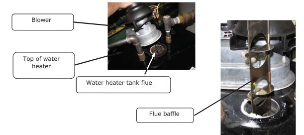
Step 6. Remove the blower from the top of the water heater.
