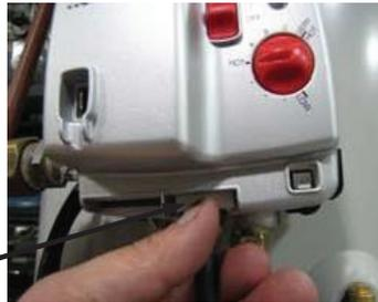
Step 3. Using a multi-meter set to the ohms setting, measure the resistance of the flammable vapor sensor.
