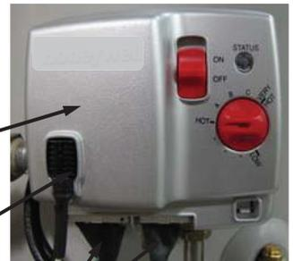
Step 7. Spin the gas control out of the water heater tank.
