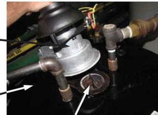
Step 8. Clean any debris from the jacket head of the water heater.
