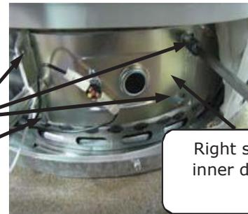
Step 6. Disconnect the pilot tube using a 7/16" wrench and the main burner feedline with a 3/4" wrench from the gas control.
