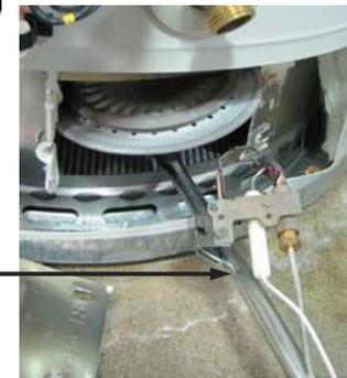
Step 9. Thoroughly inspect the burner surface area and burner port area and remove any loose debris.
