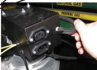
Step 6. Carefully pull out and lower the blower junction box cover.
