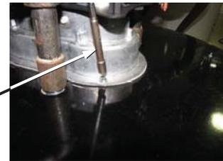
Step 7. Remove the blower from the top of the water heater.
