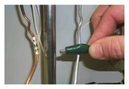
Step 4a. **For White Rodgers Mechanical:** to replace the igniter, disconnect the white (orange) wire from the igniter. Use a flat-head screwdriver under the igniter and gently pry bracket from the front of the gas calce and unhook the bracket from rear of the gas valve.
