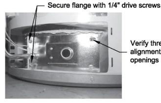
Verify threaded hole alignment with slotted openings in inner door
