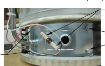
Resettable thermal switch wire connection
