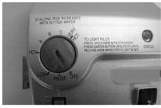
Rotate knob counter-clockwise to the "OFF" position
