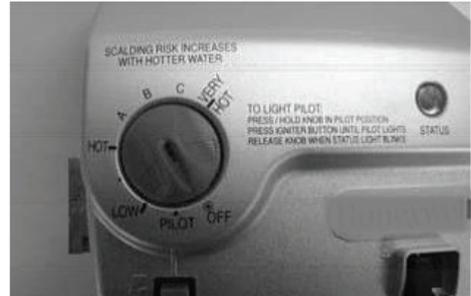
Rotate knob counter-clockwise to the "OFF" position
