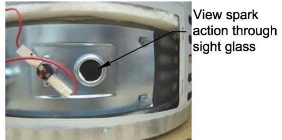
Step 3. Remove the white (or orange) wire from the gas control's igniter wire. Hold the igniter lead from the gas control to an unpainted surface such as the feedline and depress the igniter. If there is a spark, the igniter is O.K.. Otherwise, the igniter is not functioning and the pilot assembly must be replaced. See Service Procedure VI.
