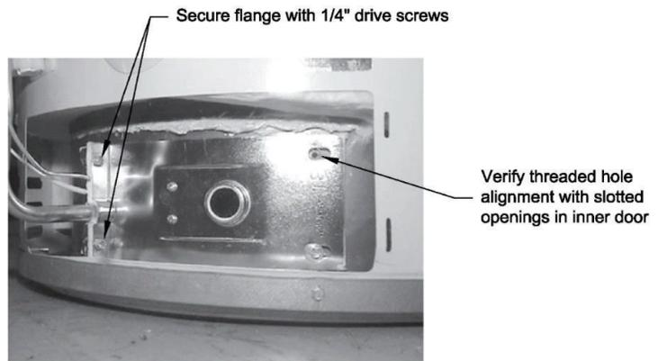
Step 10. Reconnect two (2) red wire leads from pilot assembly and gas control to resettable thermal switch.
