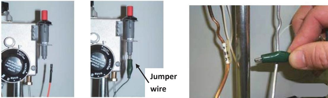
Step 4a. **For White Rodgers Mechanical:** to replace the igniter, disconnect the white (orange) wire from the igniter. Use a flat-head screwdriver under the igniter and gently pry bracket from the front of the gas calce and unhook the bracket from rear of the gas valve.
