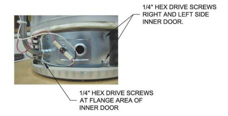
Step 7. Fully inspect inner door gaskets for the following:
