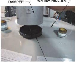
WATER HEATER TANK FLUE
