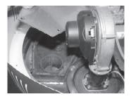
Step 8. Photo 44 shows heater with collector cover removed allowing access to anode rods and flue baffles.
