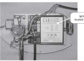
Ignition Module located on control panel
