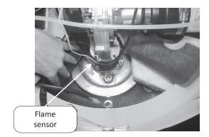
Step 8. Install new flame sensor with new gasket provided using screws from step 6. Arrange flame sensor with hook towards burner.
