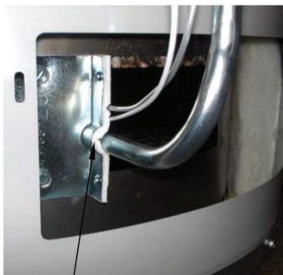
RADIUSED CHANNEL FOR FEEDLINE
