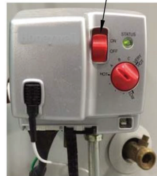
GAS CONTROL SHOWN IN THE "OFF" POSITION
