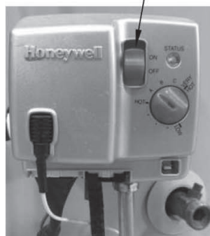
GAS CONTROL SHOWN IN THE "OFF" POSITION
