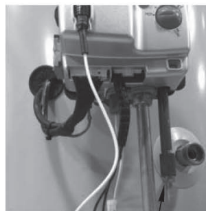
PRESSURE TAP SHOWN INSTALLED
