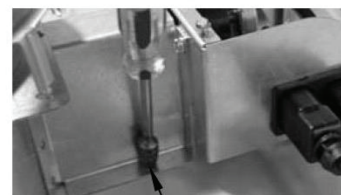
1/4" NUT DRIVER — DAMPER — TOP OF WATER HEATER
