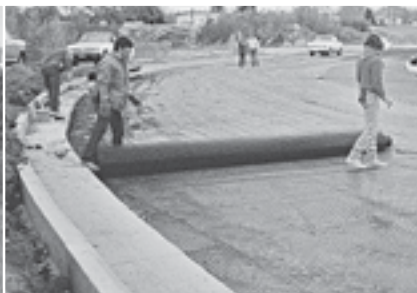
Image 5 Placing Geogrid to accommodate curves.
