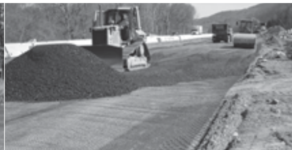
Image 9b Spreading aggregate fill over Tensar Geogrid.
