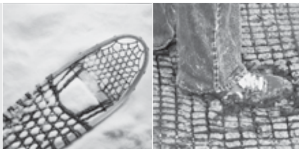
Image 1 The Snowshoe Effect – Tensar TriAx and BX Geogrids distribute heavy loads over soft soils just like a snowshoe supports the weight of a man over soft snow.
