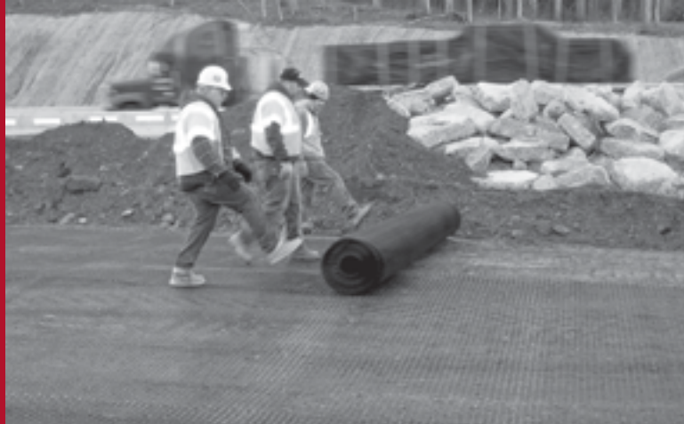
Image 3 Rolling out Tensar Geogrid.
