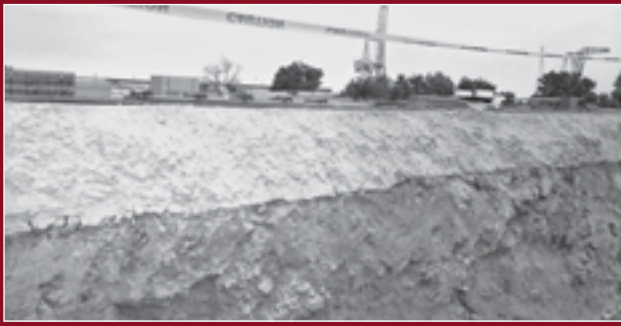
Image 13 A backhoe excavation through Tensar Geogrid.
