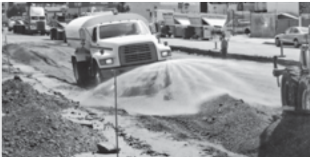
Image 10 Moistening the fill before compaction.
