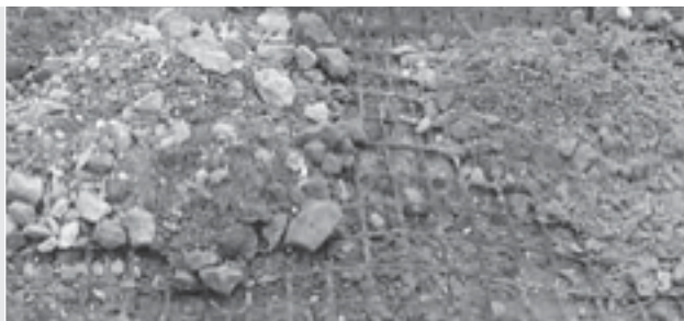
Image 7a Anchoring geogrid with piles of aggregate.
