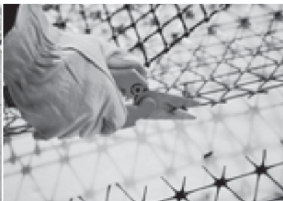
Image 6 Cutting Tensar TriAx® Geogrid is easily achieved.
