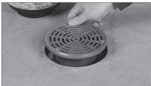
Install Finish Fixture
