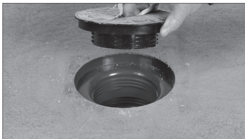
Remove Coring Plug
