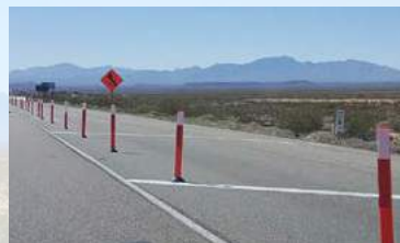
ABS Base and Posts Designed and Tested to 50 Impacts at 35 mph
