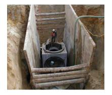
ASTM C478 sanitary sewer manhole bases with integrally cast precast inverts
