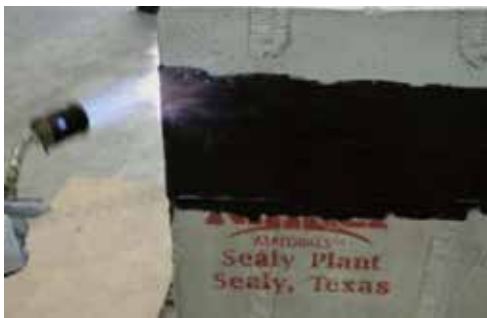
RISER-WRAP® SQUARE VAULT APPLICATION
