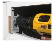
2) Screw the post into the pilot hole with the larger, #8 x 1" screw packaged with the false front kit.
