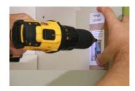
2) For a ½" overlay door, rest the door on the hinge locator block and screw the hinge to the cabinet frame. Use the ¾" washer-head screws.
