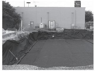
Place non-woven geotextile over prepared soils and up excavation walls. Install underdrains if required.
