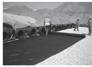
Install manifolds and lay out woven scour geo textile at inlet rows [min. 12.5 ft (3.8 m)] at each inlet end cap. Place a continuous piece (no seams, double layer) along entire length of Isolator<sup>®</sup> Row(s).
