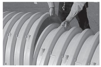
Continue installing chambers by overlapping chamber end corrugations. Chamber joints are labeled "Lower Joint – Overlap Here" and "Build this direction – Upper Joint" Be sure that the chamber placement does not exceed the reach of the construction equipment used to place the stone. Maintain minimum 6" (150 mm) spacing between rows
