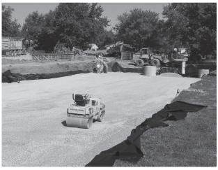
Place clean, crushed, angular stone foundation 6" (150 mm) min. Compact to achieve a flat surface.
