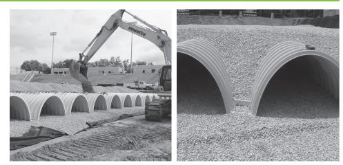
No equipment shall be operated on the bed at this stage of the installation. Excavators must be located off the bed. Dump trucks shall not dump stone directly on to the bed. Dozers or loaders are not allowed on the bed at this time.
