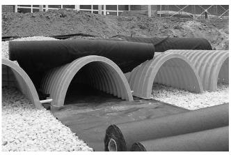
Place two continuous layers of ADS Woven fabric between the foundation stone and the isolator row chambers, making sure the fabric lays flat and extends the entire width of the chamber feet. Drape a strip of ADS non-woven geotextile over the row of chambers (not required over DC-780). This is the same type of non-woven geotextile used as a separation layer around the angular stone of the StormTech system. **2**
