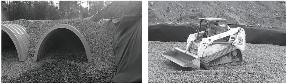
Continue evenly backfilling between rows and around perimeter until embedment stone reaches tops of chambers. Perimeter stone must extend horizontally to the excavation wall for both straight or sloped sidewalls. **Only after chambers have been backfilled to top of chamber and with a minimum 6" (150 mm) of cover stone on top of chambers can small dozers be used over the chambers for backfilling remaining cover stone.**
