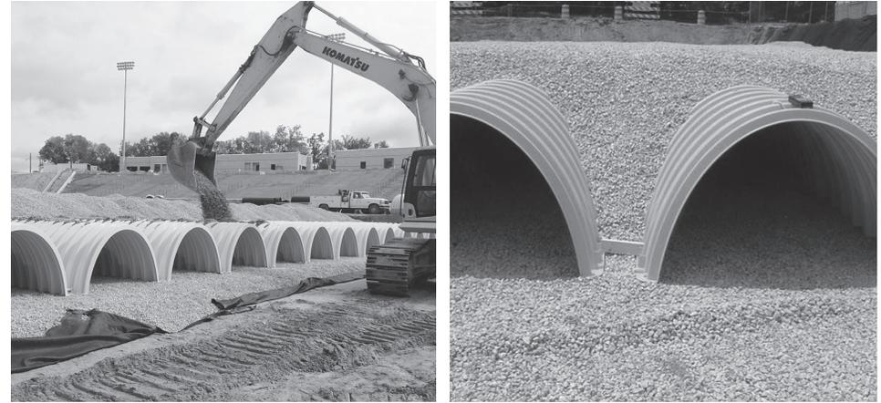
No equipment shall be operated on the bed at this stage of the installation. Excavators must be located off the bed. Dump trucks shall not dump stone directly on to the bed. Dozers or loaders are not allowed on the bed at this time.
