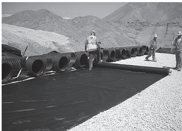
Install manifolds and lay out woven scour geo textile at inlet rows [min. 12.5 ft (3.8 m)] at each inlet end cap. Place a continuous piece (no seams, double layer) along entire length of Isolator® Row(s).
