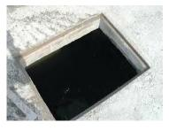
Grate removed and prepared for installation of the Grate Inlet Skimmer Box.
