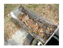
Standard Capacity Curb Inlet Basket removed from shelf inside inlet. The filtration basket holds dried debris ready for disposal.
