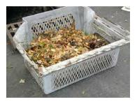
Grate Inlet Skimmer Box filtration basket removed by hand for manual disposal of debris and basket cleaning.
