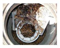
High Capacity Curb Inlet Basket after storm event containing dry foliage and debris ready for collection and disposal.
