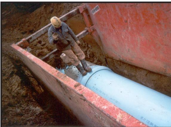
the pipe lengths in proper alignment. Brace the bell while the spigot end is pushed through the gasket so that previously completed joints in the line will not be “stacked,” “over belled,” or inserted past the second reference mark. (refer to Encasements.) Push the spigot end in until the lip of the bell is between the reference marks on the spigot end. If the spigot is inserted beyond the first insert reference mark, laying length will be lost. Loss of laying length
