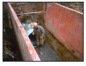
of over excavation and bedding for 48" -60" nominal diameter pipes. The bedding should consist of an evenly graded, free flowing, granular material which is free of large stones or frozen material and with particle size of up to approximately 10% of the pipe size and no larger than 1  $\frac{1}{2}$ " in size. Bell holes should be utilized to reduce axial deflection and support the barrel of the pipe.
