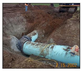
Foundation: An adequate or stable foundation should be present (or provided) to uniformly support the full length of the pipe. Bell holes should be provided at each joint to permit proper assembly and support of the pipe. Unstable trench bottoms shall be stabilized by methods and with materials required, by the specifying engineer, to provide adequate and permanent support for the conditions encountered.
