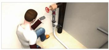
The In-line Pitotless Nozzle in a stairwell standpipe test.
