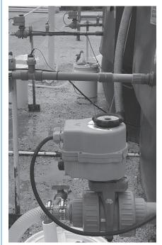
Industrial TUBV with Electric Actuators on a chlorine dispensing system in Florida.
