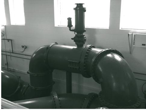
Air Valves are commonly found in plant service as well as pipelines for efficiency and protection. The model shown above is a 48A/308 with flanged outlet and optional Cam-Centric® Plug Valve for isolation and maintenance.
