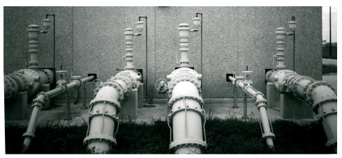
Surge-Suppression Air Valves and Isolation Valves in a pump discharge application.
