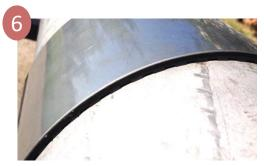
Allow the gasket to fully compress, and recheck the studs tightness. It is important to re-torque Tapped Repair Clamps when used as a "hot tap" saddle after the tap has been made.
