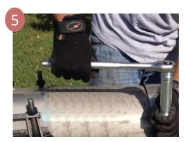
Evenly tighten the studs working from the center outward. Maintain an even gap between fingers studs when installing multi-panel repair clamps.
