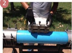
Loosen nuts to the end of the stud, place the clamp around the pipe centered over the break or damage area with the gasket flap at the top.
