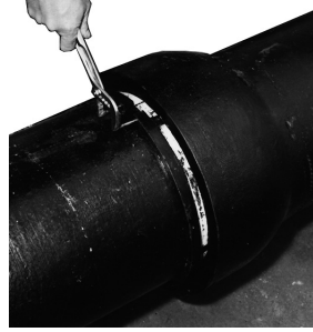
DISASSEMBLY OF 4"-12" FLEX-RING
