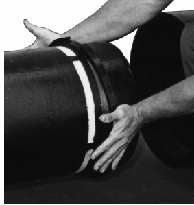
FIELD ASSEMBLY OF FLEX-RING
