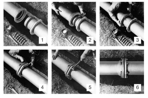
1. Thoroughly clean socket and plain end of all rust or foreign material; slip the gland over plain end with the lip extension toward plain end, followed by the gasket with thick section facing the gland. Gaskets to be installed during very cold weather should be warmed first.\*
